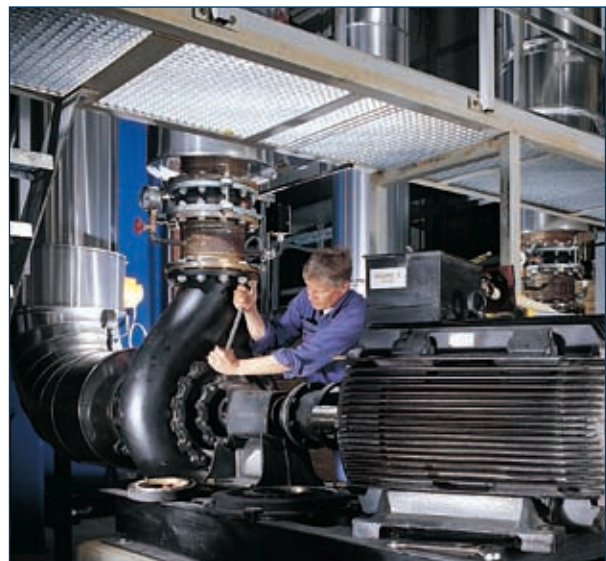
NK pump in district heating plant.
