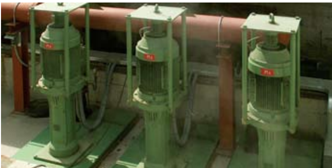
Vertical PEMO pumps for transfer of slurries
