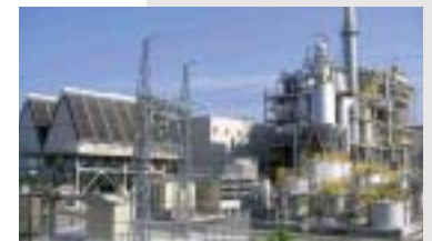
Hita Power Plant, Hita Wood Power Co., Ltd. Using ligneous biomass as a material, ICFB recovers heat. This commercial biomass power plant generates 12 MW of power with a steam turbine.
