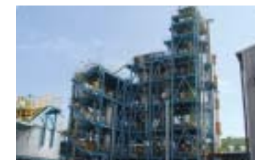
Pressurized two-stage gasification system EBARA and Ube Industries, Ltd. have jointly developed a chemical recycling system that collects ammonia from waste plastic by applying waste gasification technology.
