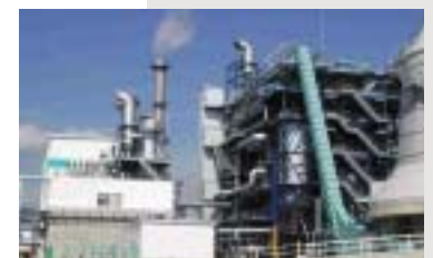
Nakoso Plant Biomass Boiler, Nippon Paper Group, Inc. This facility has a processing volume of 514 t/d, and generation capacity of 15 MW. The facility recovers heat using mainly wood chips from construction waste, and generates power with a turbine for energy for use in the plant.
