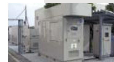
Micro gas turbine cogeneration package for digestion gas application
