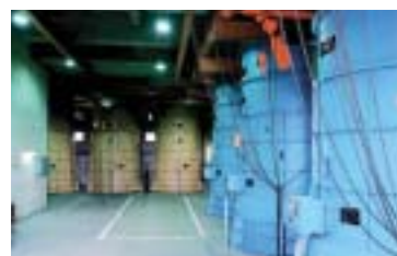
Axial fan for the Tokyo Bay Tunnel ventilation facility
